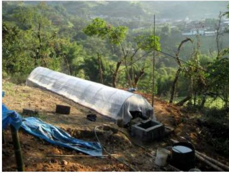
Figure 5.8 – A common tubular digester configuration with a clear plastic cover used in South America (Galvin, 2013).
